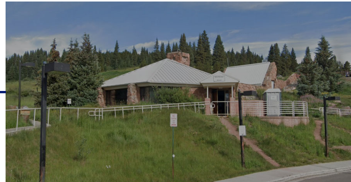
Current Rest Area Site and Building
